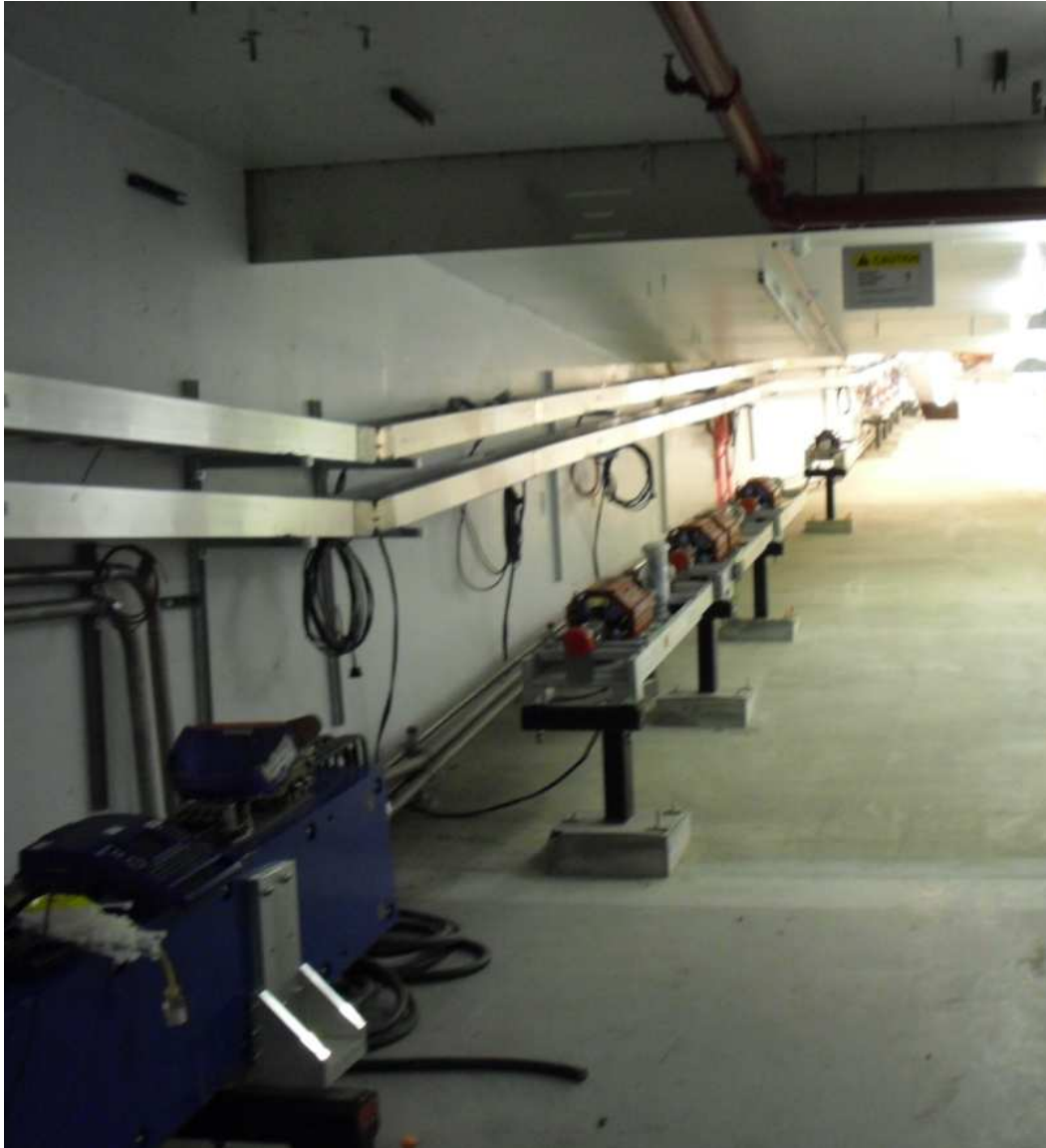
Tagger Transport girders
